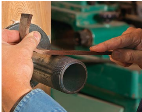
Create the next bend. Being careful not to reheat the first bend, work on bending the second section.
